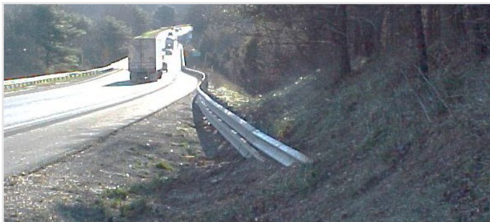
Source: FHWA Roadside Safety Systems Design, Inspection and Maintenance Training
